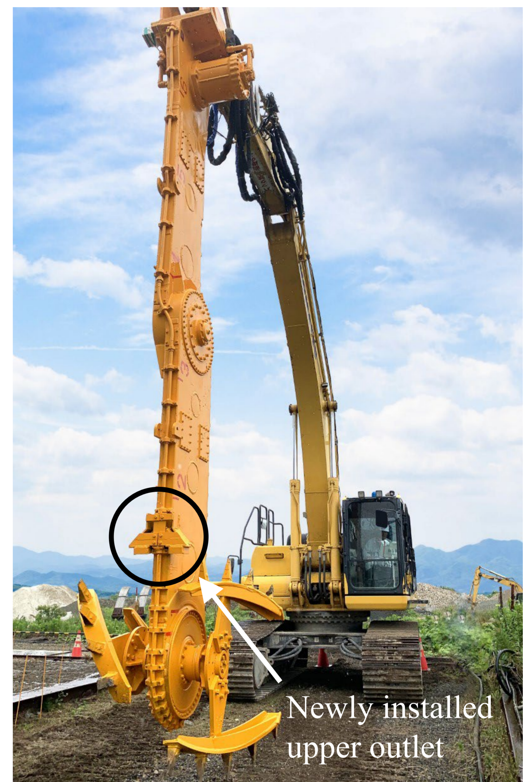
Construction machine of WILL-m method
