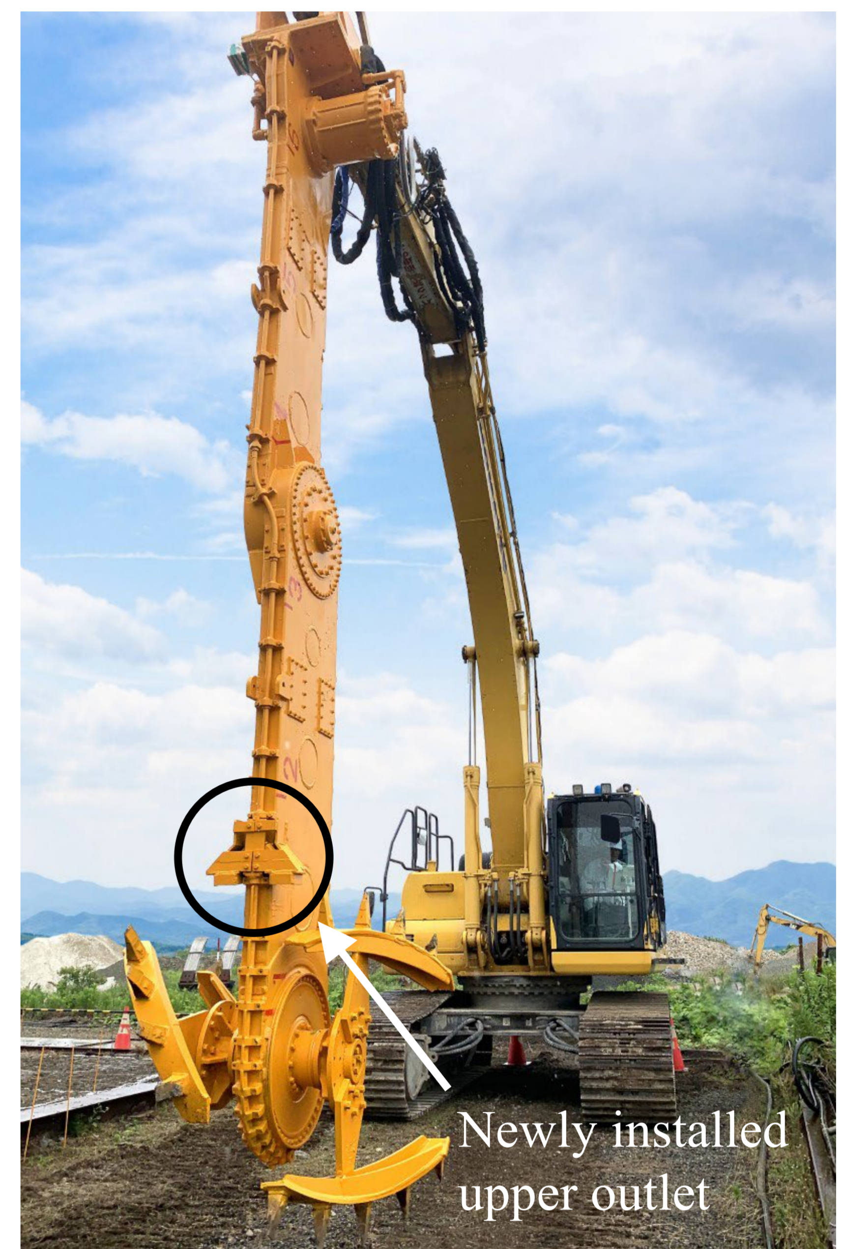
Construction machine of WILL-m method
